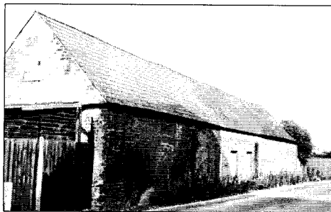
The rear of the stables before they were demolished. Photo: Eve Durnall, 14th August 1988
